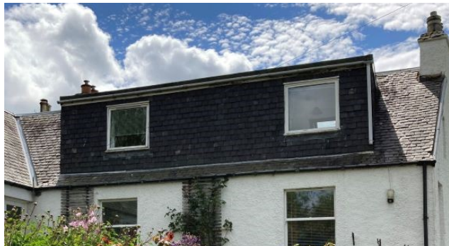
Figs. 54 and 55: over-scaled non-traditional dormer, and poor quality repairs to stone
