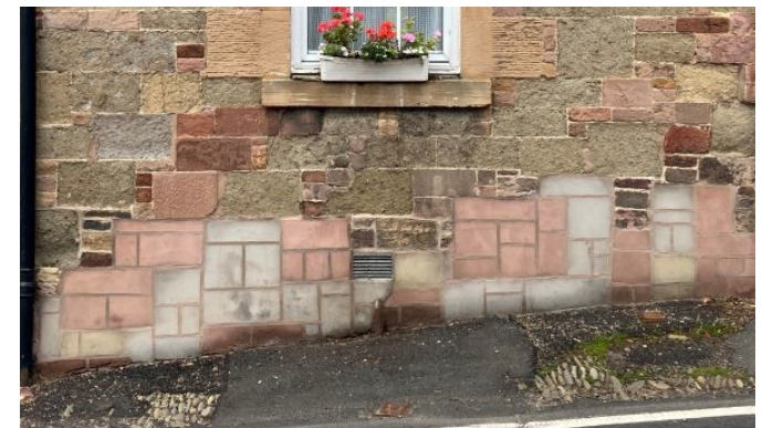
Figs. 54 and 55: over-scaled non-traditional dormer, and poor quality repairs to stone
