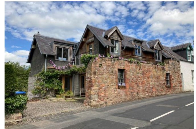
Fig. 30 (top): Eildon Housing Association development by Walter Wood Associates responds to the topography and urban grain of the area whilst using traditional forms and detailing
