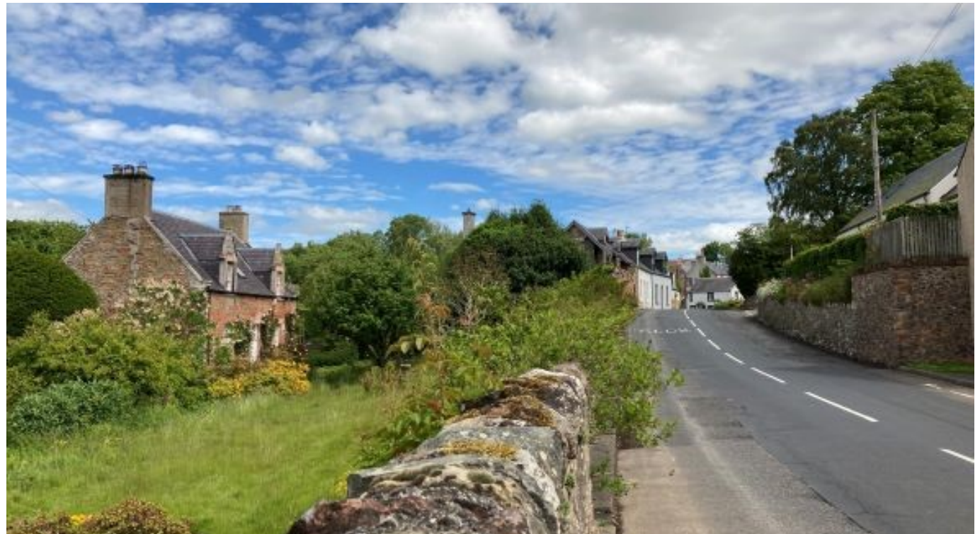
Fig. 1: Main Street, looking east with Saugh Cottage to the left
